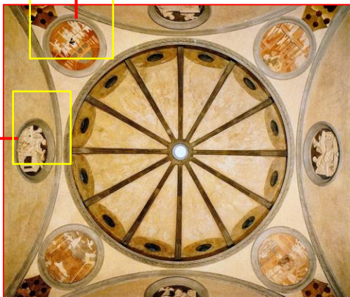
Umbrella dome: Stone radial ribs.
